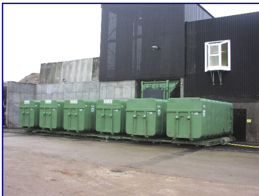
Traversing shifting system in front of a transfer station
